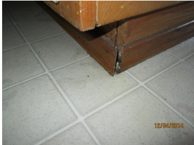
Backside of panel showing unpainted water damage in side cabinet in kitchen. The warped water damaged base molding on kitchen cabinet is shown above right.
