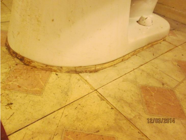
Toilet not seated properly. Bathroom sink cabinet has past water damage, needs replacement.
