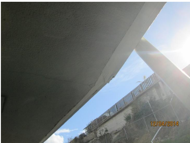
Roof above second story walk way showing eave and fascia water damage and rot.
