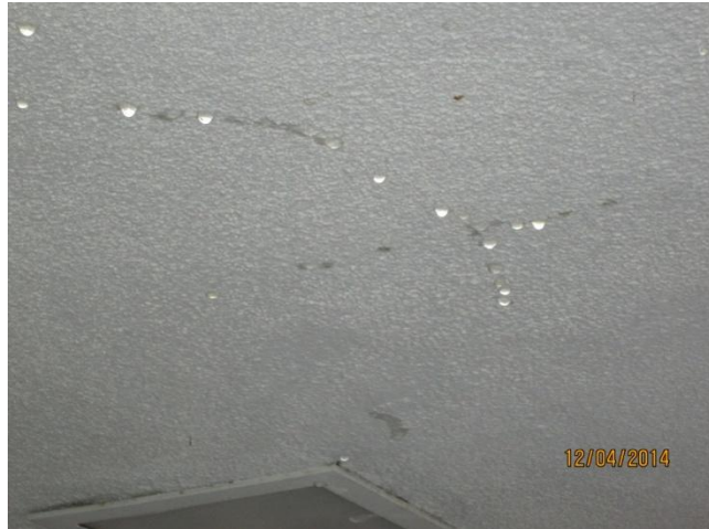
Results of water entering cracks on second story balcony walkway and dripping through the soffit area, stucco to the sidewalk in the main traffic area below.
