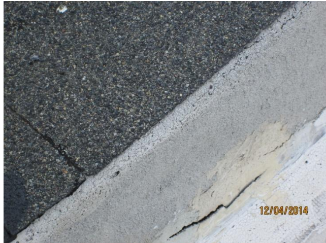
Additional areas of compromised water proofing above laundry room and water heater room.
