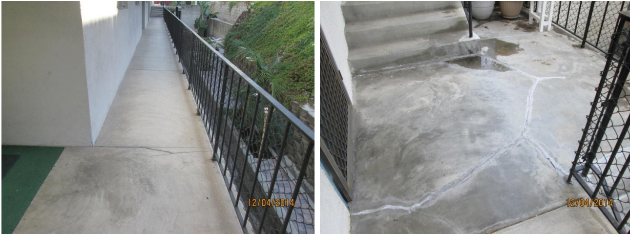
Upstairs balcony walkway with surface cracks that allow water into structure and is damaging the soffit area below.
