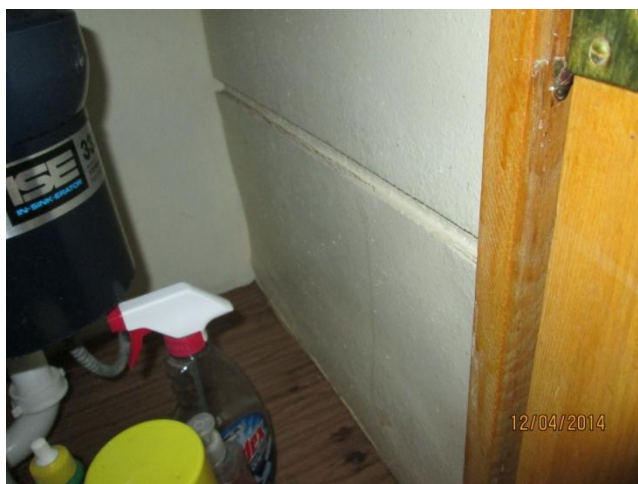
Kitchen ceiling has repaired crack in the same direction as living room crack. The sink cabinet has past water damage and the damaged cabinet side wall panel has been painted.
