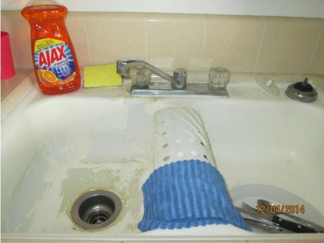
Kitchen sink in poor condition needs replacement.
