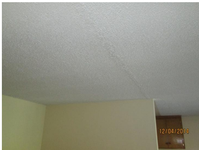
Ceiling of living room has a repaired but visible crack that runs the width of the room.
