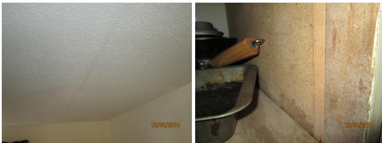
Living room ceiling has repaired crack running length of the room. Kitchen sink cabinet has past water damage to interior. No elevated moisture levels present.
