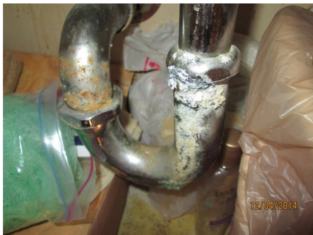
Under sink in bathroom elevated moisture levels and poor drain pipe condition appears to be leaking.
