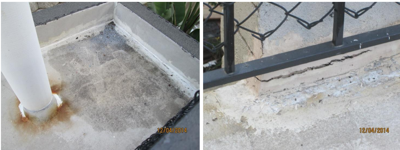
Compromised water proofing above laundry room and water heater room.
