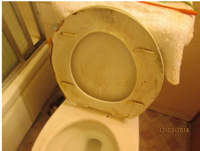
Elevated moisture levels on drywall next to tub and around angle stop evidence of patched wall repair work. Surface mold growth in bathroom especially on toilet seat and fixture. High humidity in bathroom and unit.
