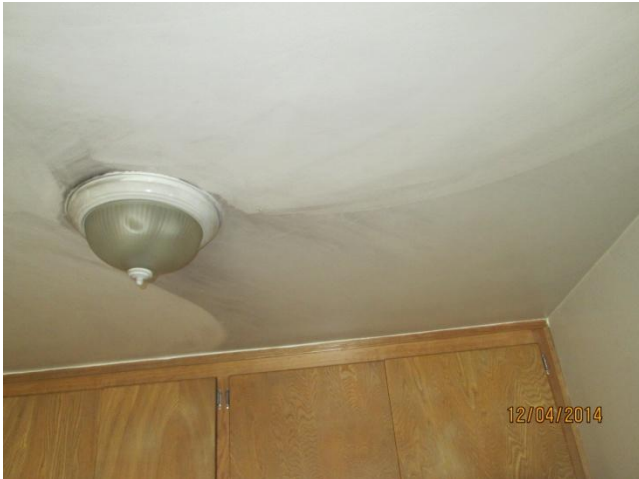
Additional view of other area of smoke damage in kitchen. No other issues noted in this unit.
