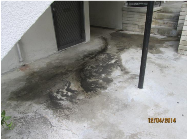
Results of water entering cracks on second story balcony walkway and dripping through the soffit area, stucco to the sidewalk in the main traffic area below.
