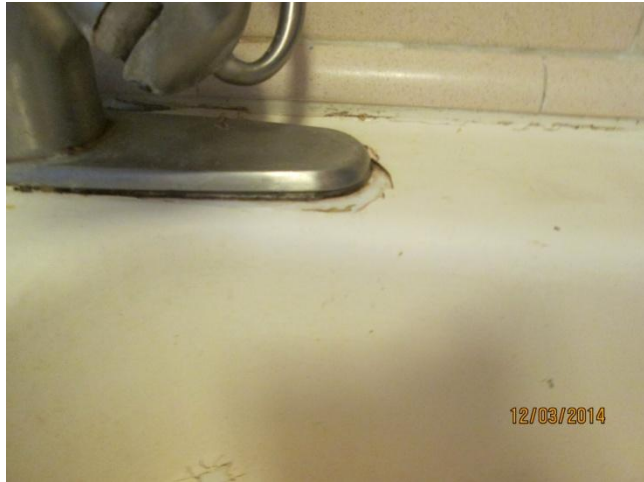
Kitchen sink refinishing is delaminating as seen at fixture bottom edge.
