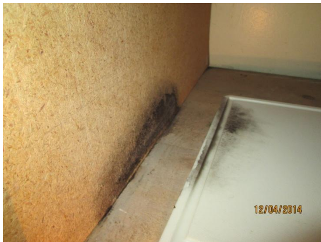
Kitchen sink in poor condition. Sink cabinet has water damage and visible mold.
