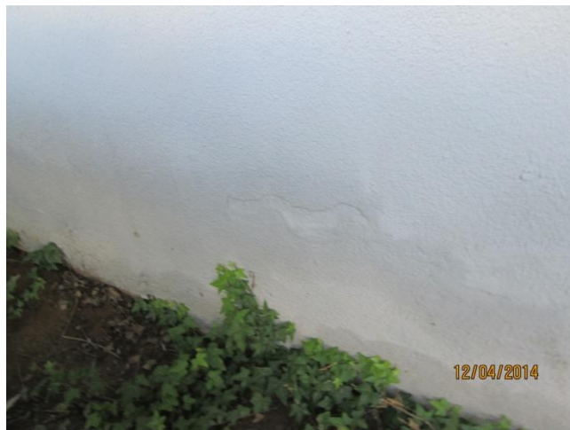
Above photos show stucco damage, spall and blistering from excess ground moisture wicking into the stucco material due to lack of weep screed installed at the stucco wall.
