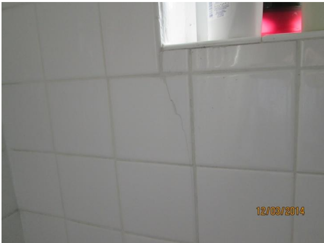
Cracks in tile surround for tub, elevated moisture levels in wall between tub and angle stop.
