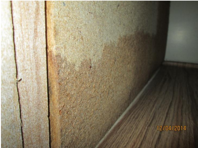
Backside of panel showing unpainted water damage in side cabinet in kitchen. The warped water damaged base molding on kitchen cabinet is shown above right.
