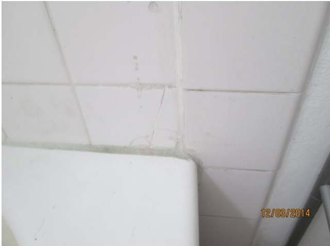
Cracked tiles, lacking caulk seal at fixtures.
