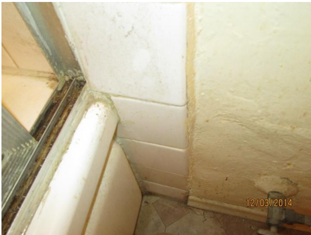
Elevated moisture levels on drywall next to tub and around angle stop evidence of patched wall repair work. Surface mold growth in bathroom especially on toilet seat and fixture. High humidity in bathroom and unit.
