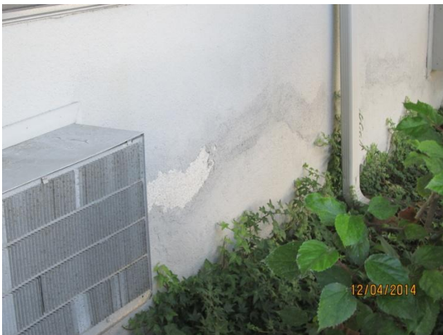
Above photos show stucco damage, spall and blistering from excess ground moisture wicking into the stucco material due to lack of weep screed installed at the stucco wall.
