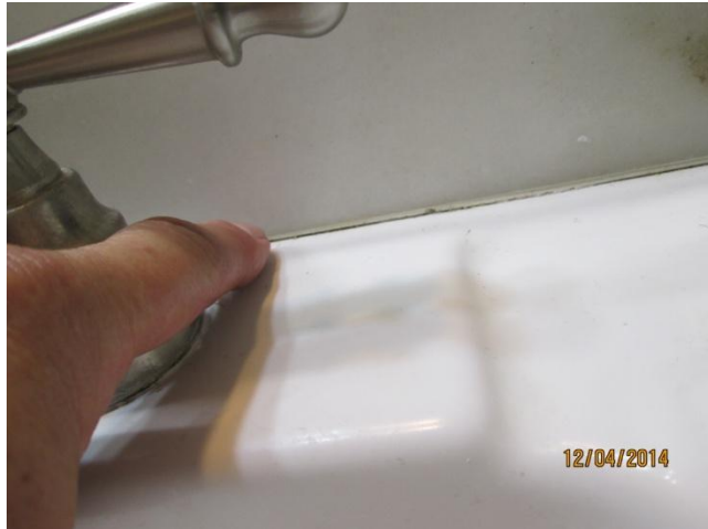
Bathroom sink cabinet shelf has elevated moisture levels due to lack of good caulk seal at rear of sink.
