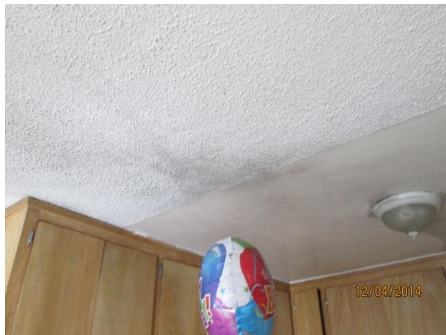
Kitchen ceilings and cabinet exteiors affected by smoke damage from previous fire event.
