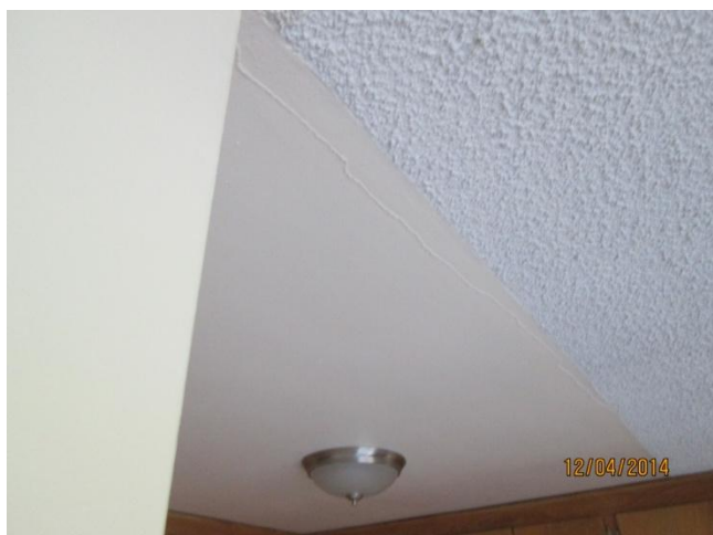
Kitchen ceiling has repaired crack in the same direction as living room crack. The sink cabinet has past water damage and the damaged cabinet side wall panel has been painted.
