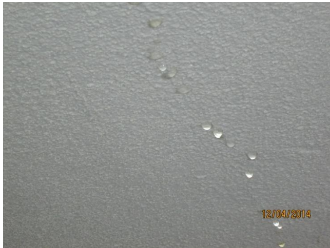
Water heater room ceiling is wet as shown by the meter readings. Entire ceiling is water stained.
