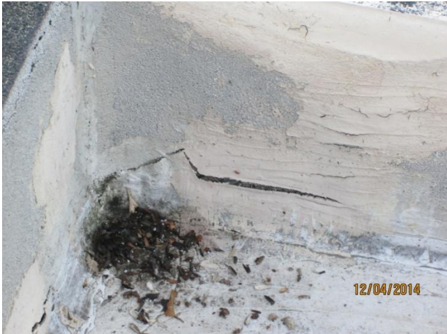
Additional areas of compromised water proofing above laundry room and water heater room.
