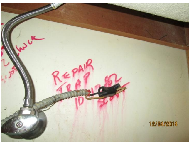
Under kitchen sink revealed dangerous wire situation. Former water damage stains remain in cabinet side panels and bottom shelf. These are dry now.
