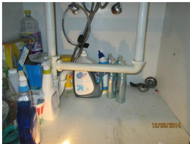
Former leak into sink cabinet now dry, some damage to cabinet side panel shelf has been replaced.
