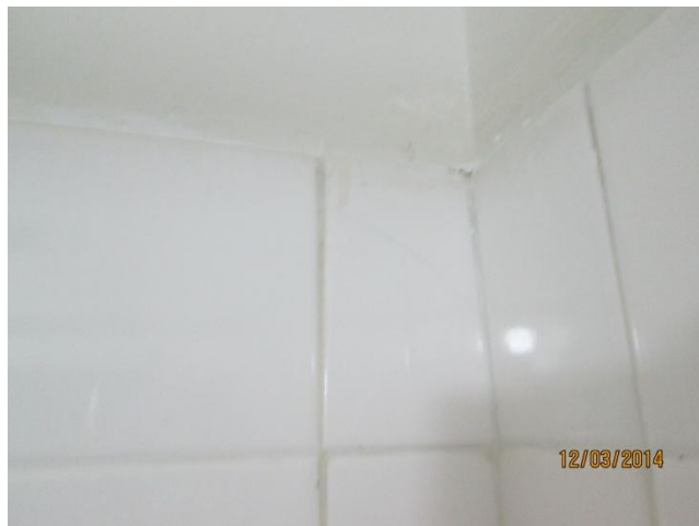
Bathroom shower enclosure tile has cracks; some tile in field is buckling, moisture levels could not be measured as tiles were wet.
