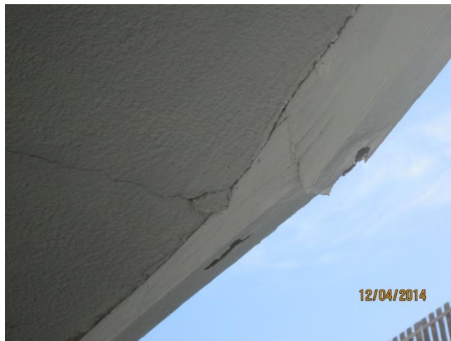
Roof above second story walk way showing eave and fascia water damage and rot.
