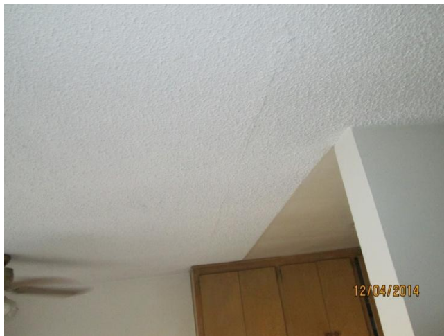
Elevated moisture levels going up 2' from floor to side of tub enclosure in bathroom. Dining room ceiling has repaired crack running the width of the ceiling.
