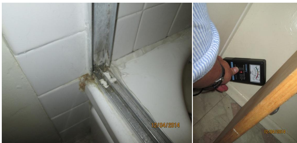
Tub to shower door seams appear to leak. Wall next to tub and behind toilet reads elevated moisture levels.
