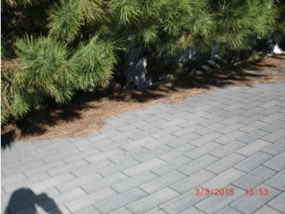
Pine tree debris on the roof at 4239.
