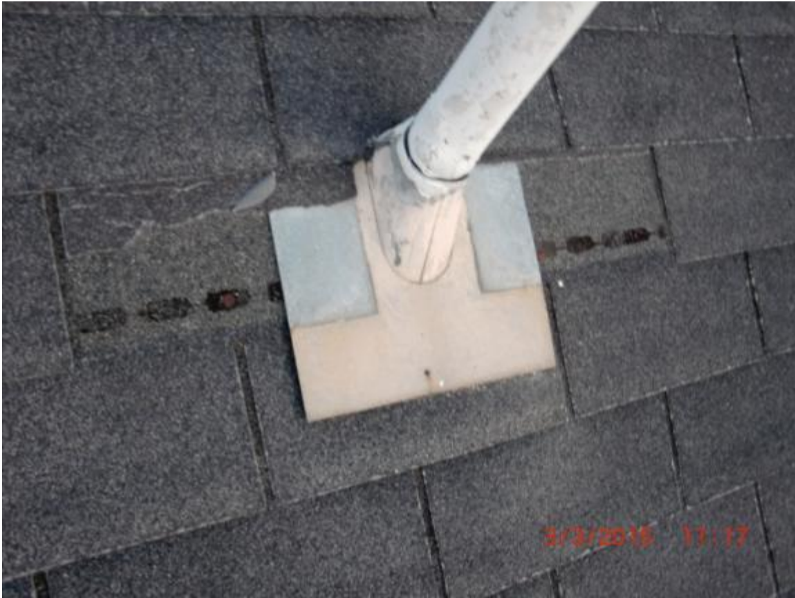
Missing shingle tabs at the south side of 4235. There was staining below this area.
