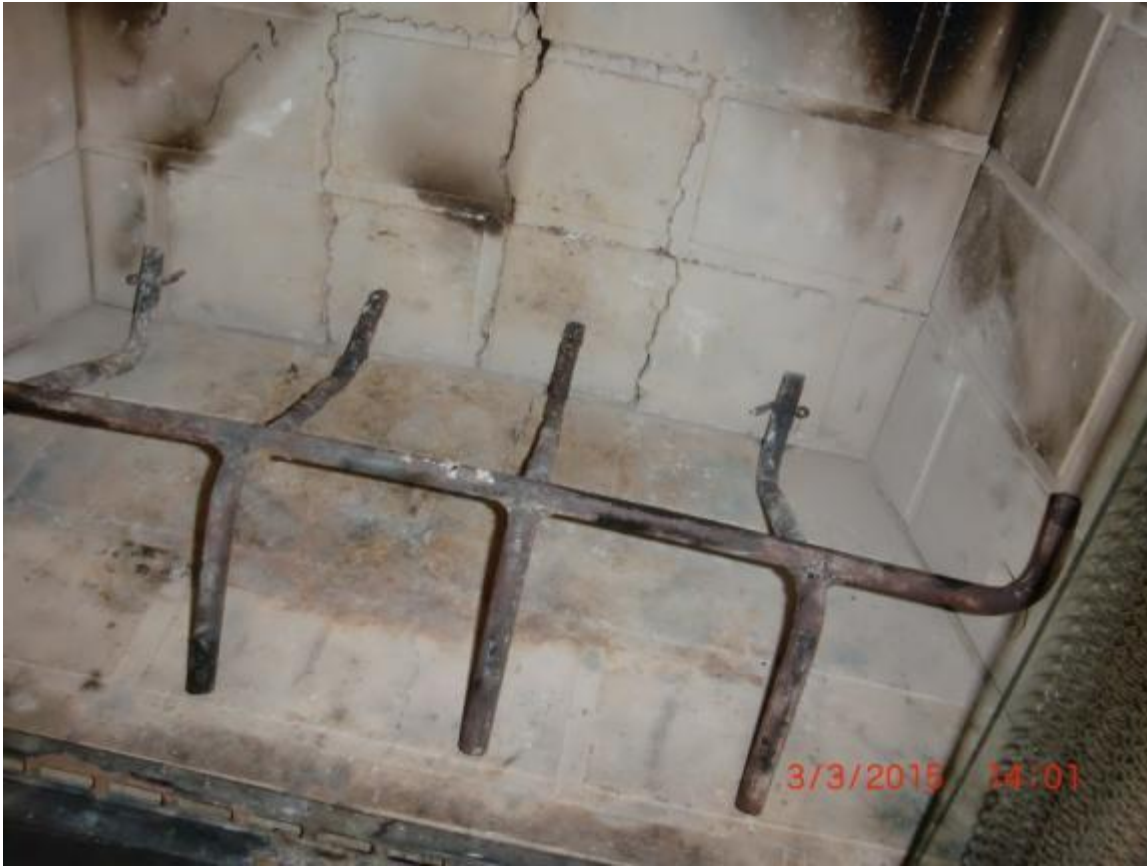
Cracking at hearth and back refractory panels at 4239#7. This is an example of cracking that is probably too far gone for the patching to hold.
