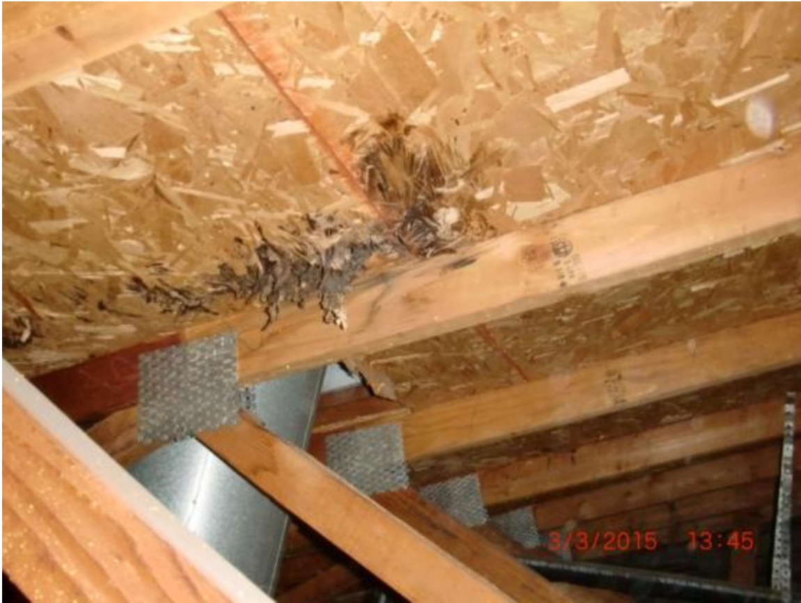
Damaged decking from roof leaks near the fireplace chimney at 4239#4. There are other soft spots in this area.
